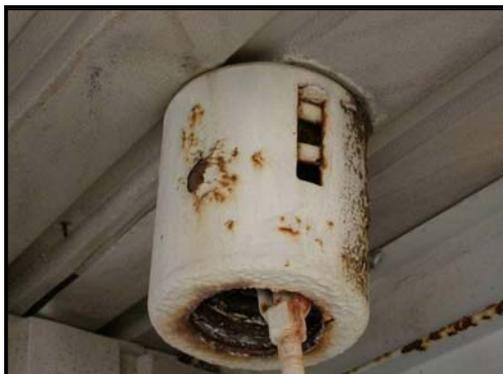
**Figure 3. Variable Support Hanger Displaying Severe Corrosion**
