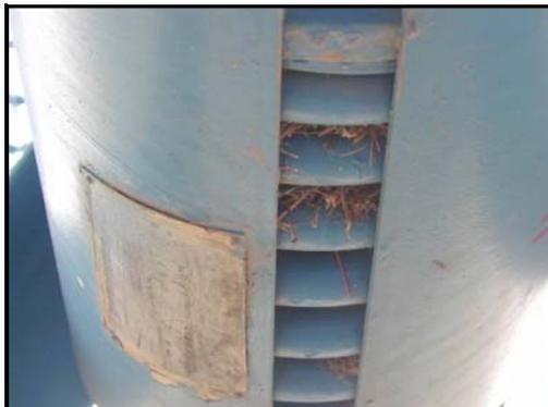
**Figure 2. Closer View of Constant Support Hanger Fouled by Nesting Birds**
