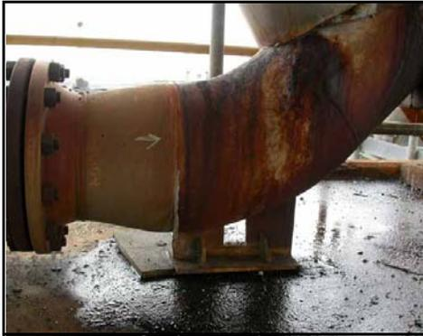
**Figure 4. Slide Plate Displays a Dislodged HDPE Pad**
