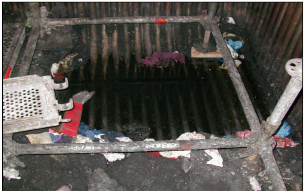
Figure 5. Decanting floor “puddle” area with smelt bed removed.
