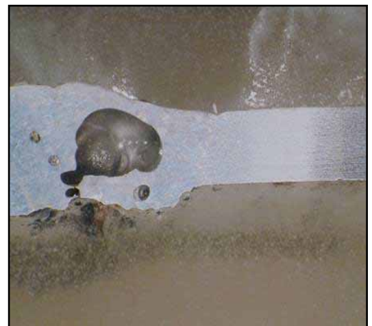
Figure 1. Example of Weld Porosity in a Superheater Weld
