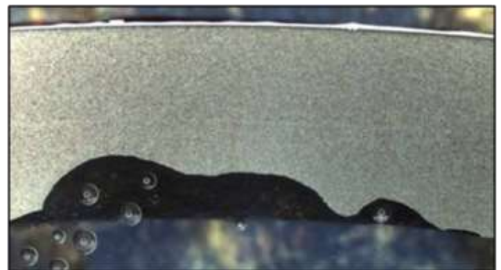
Figure 5. Photograph shows severe pitting in a cross section of the galvanized pipe.
