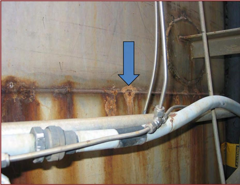
Figure 1. Close-up of leaks at first course weld.
